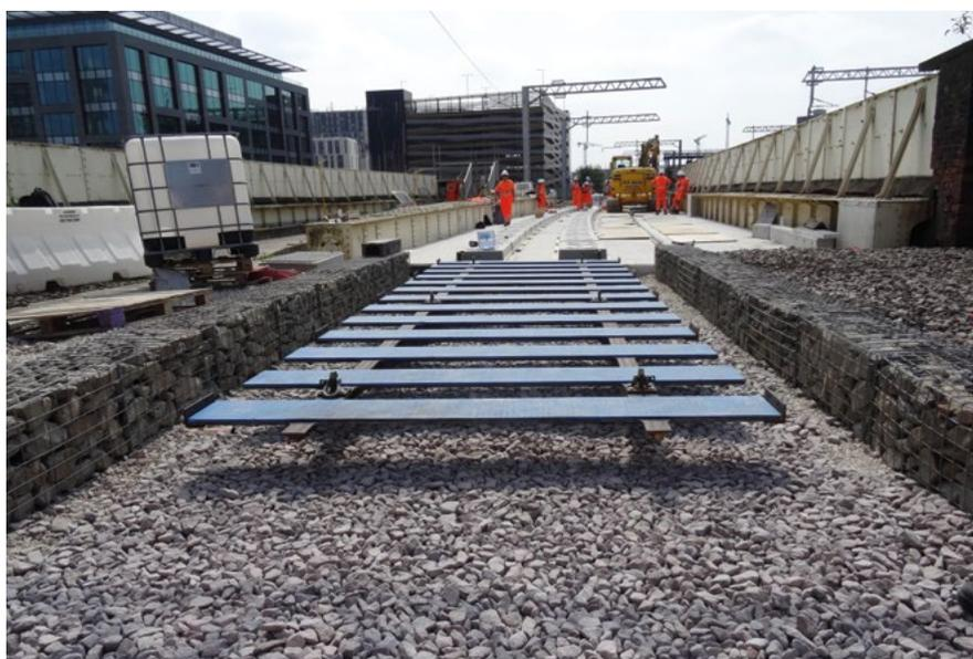
The greatest challenge during the construction phase was the core drilling of the highly reinforced deck slab. Once the IVES-elements are positioned they will be levelled and grouted with a fast-hardening grouting mortar; this fills the gaps between rail fastenings and the structural elements. Plexiglass windows ensure that a successful grouting operation with flawless surface quality has been accomplished.
