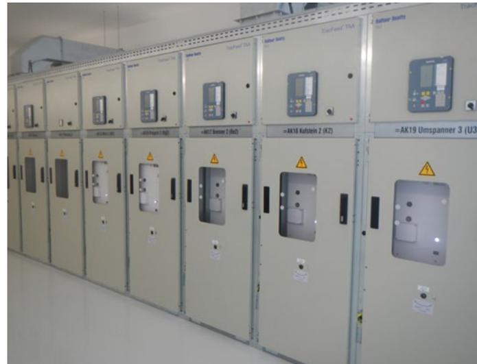
The medium-voltage interior single-phase traction-current switchgear is the "heart" of the plant.
