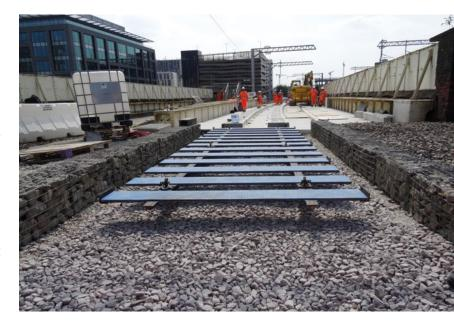
The greatest challenge during the construction phase was the core drilling of the highly reinforced deck slab. Once the IVES-elements are positioned they will be levelled and grouted with a fast-hardening grouting mortar; this fills the gaps between rail fastenings and the structural elements. Plexiglass windows ensure that a successful grouting operation with flawless surface quality has been accomplished.
