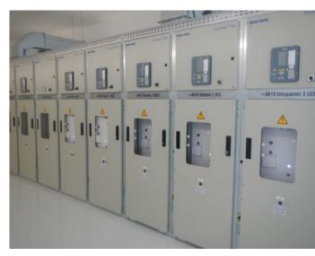
The medium-voltage interior single-phase traction-current switchgear is the "heart" of the plant.
